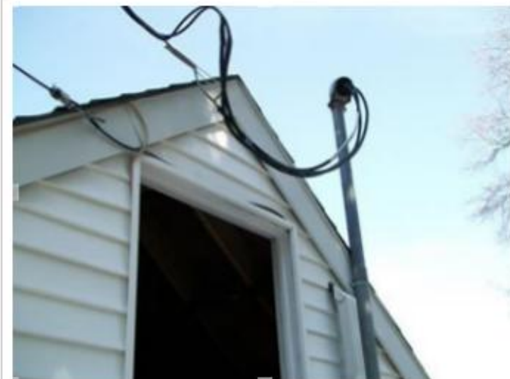
Wire clamps are widely used to support communication wires at span clamps , drive hooks and various drop attachments .
